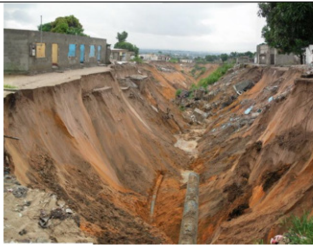
Photo 1: Initial status at the Boukeni ravine, before placing sandbags and planting vetiver
