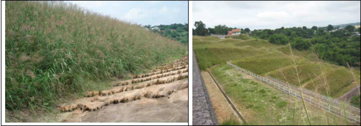
Photos 13 and 14: Same site as in photos 11 and 12 (May 2011), the vetiver hedges having prevented all erosion despite record rainfall exceeding 70 mm
