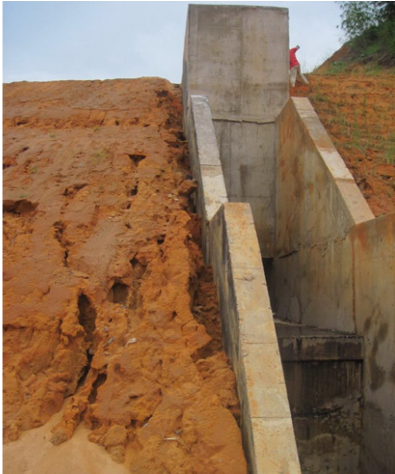
Photo 10: Damage on the slopes and embankments adjacent to the Casis drain site (Dec. 2009)
