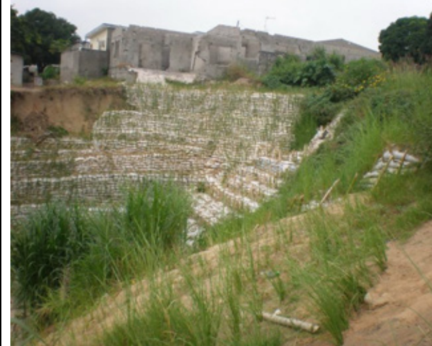
Photo 8: The Pylôn site two months after planting vetiver on parts of the site (June 2009)
