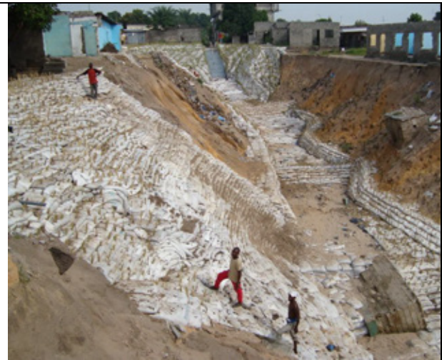
Photo 2: Placing bags containing topsoil and vetiver planting on the Boukeni site (February 2009)
