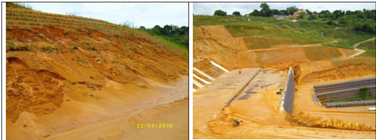
Photos 11 and 12: Damage on the slopes at the Casis site (April 2010)
