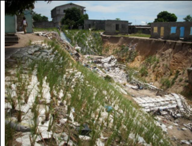
Photo 3: The Boukeni site 2 months after planting vetiver directly into the bags of topsoil (April 2009)
